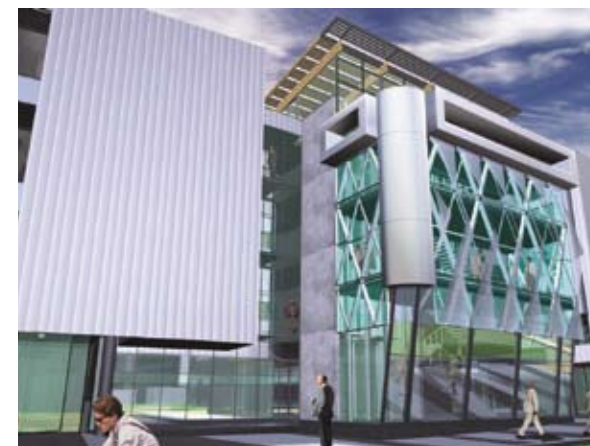
The Monash STRIP 2 building will contain more than 9800m of Crane copper tube and around 4800 Viega press-fit fittings.
